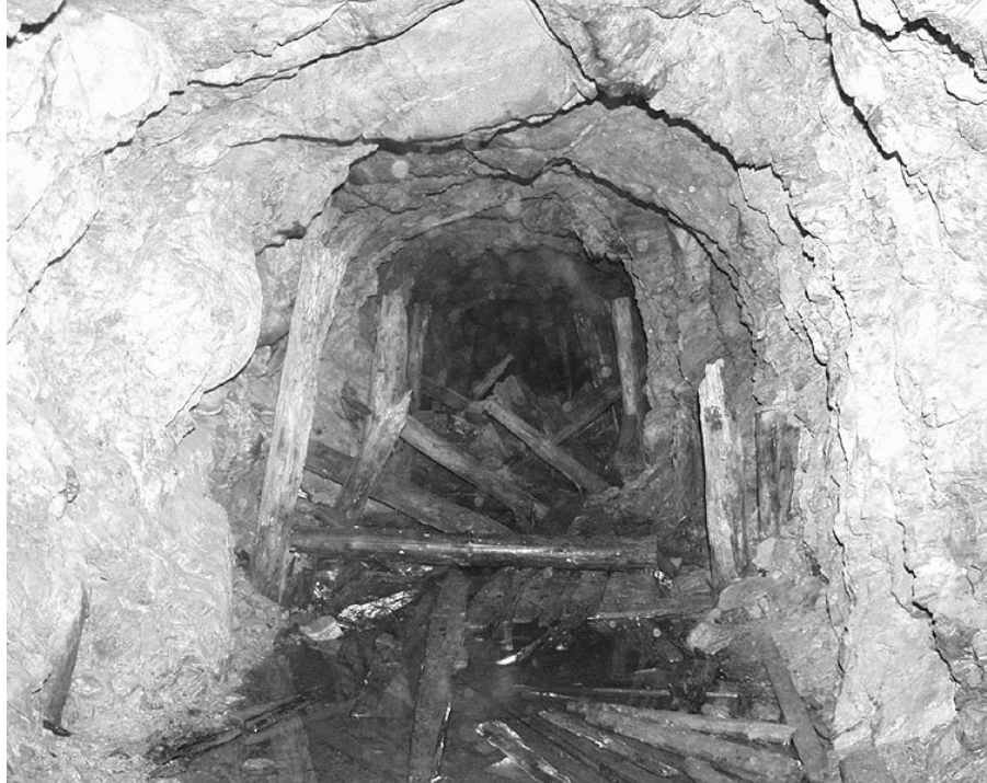
Unlined and Crumbling Tunnel Section in Wlodarz
